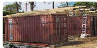
The team built trusses and erected them between our two containers. Then they put the roof on (yeah!), which was a big step.
